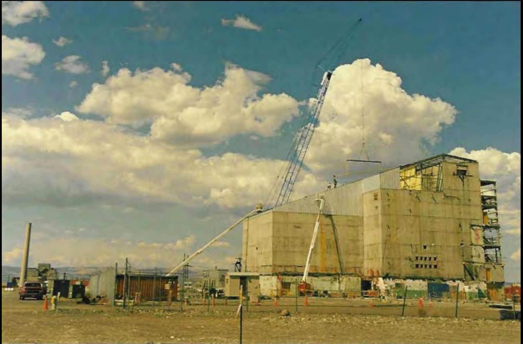
Hanford's C Reactor being cocooned
