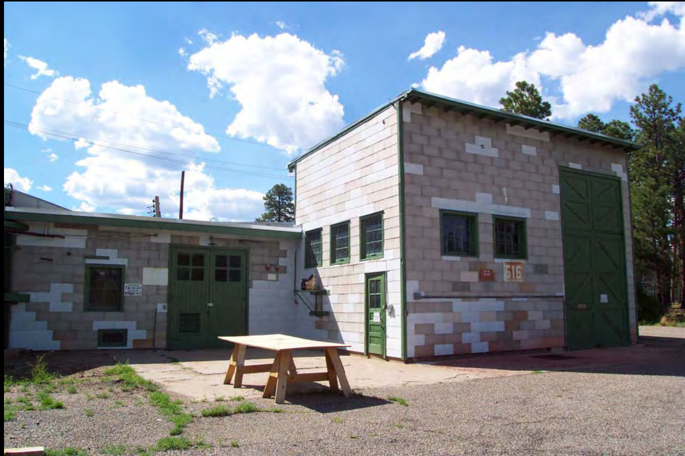
The Restored "V Site" (October 2006)
