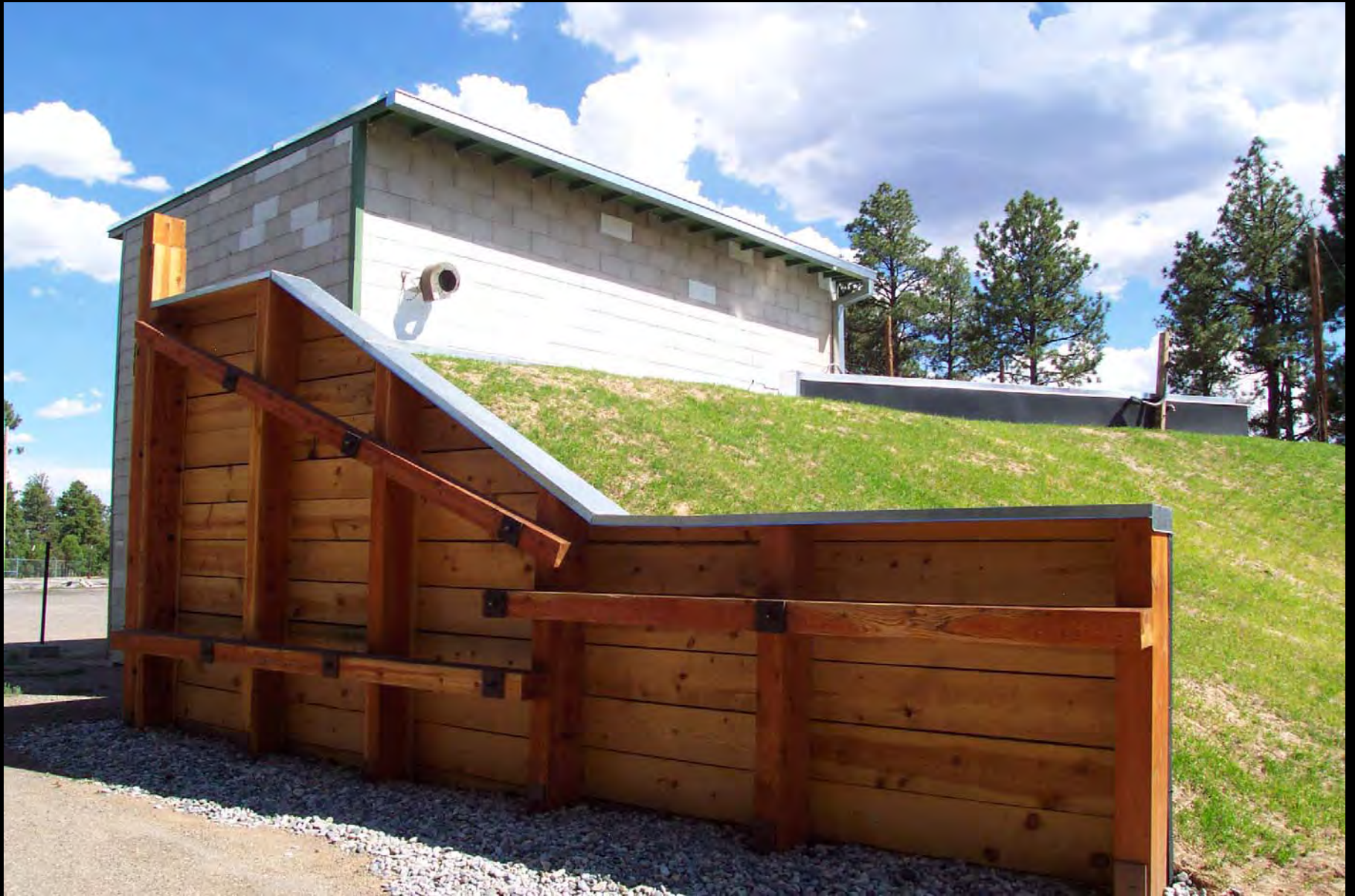
The restored retaining wall at the "V Site"
