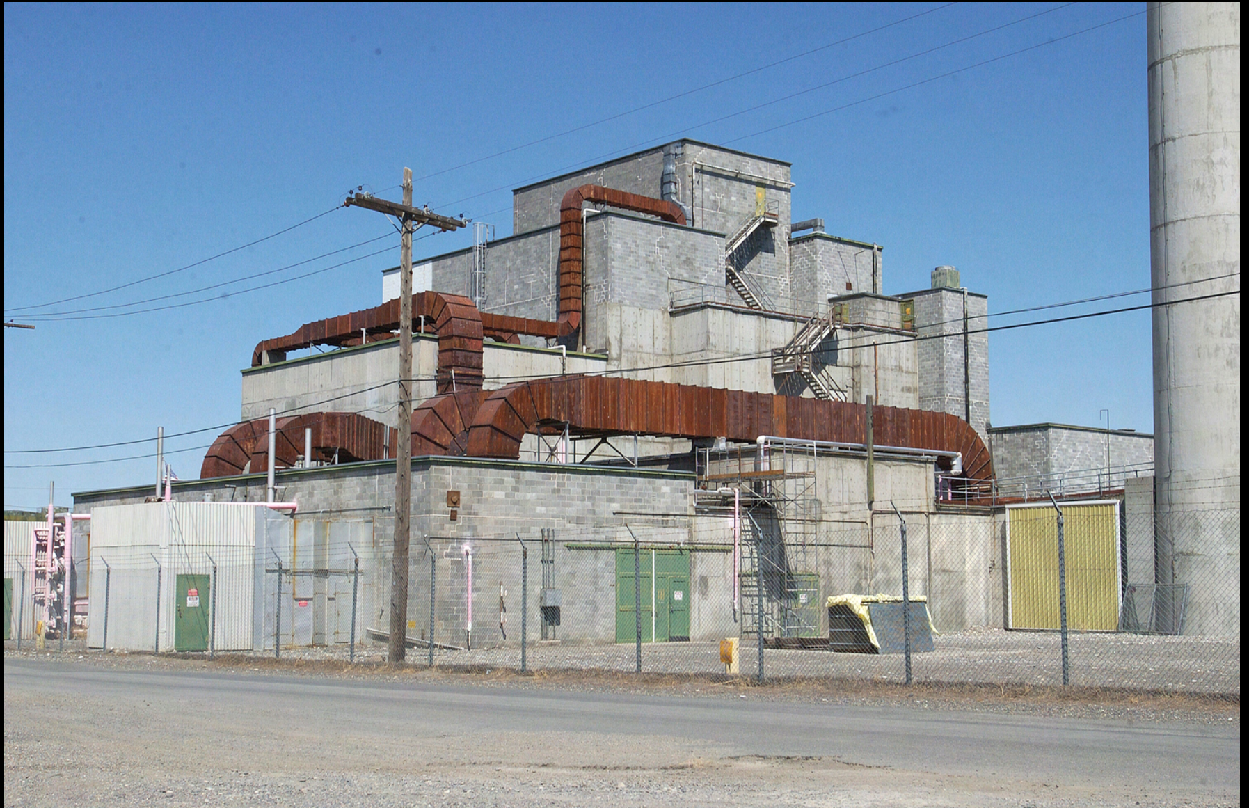
New Roof for B Reactor
